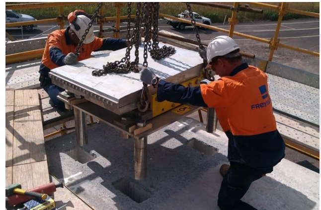
Professional bearings installation by Freyssinet teams
