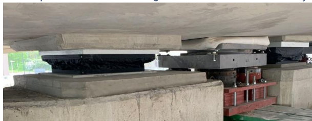
Bearing Bodygarde™ during bearing replacement works.
