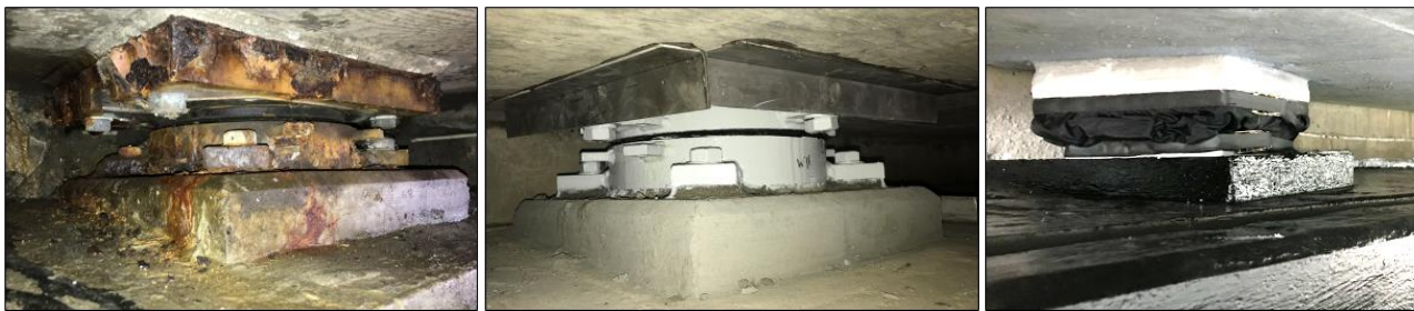
Steps of life extension of a pot bearing damaged by corrosion
